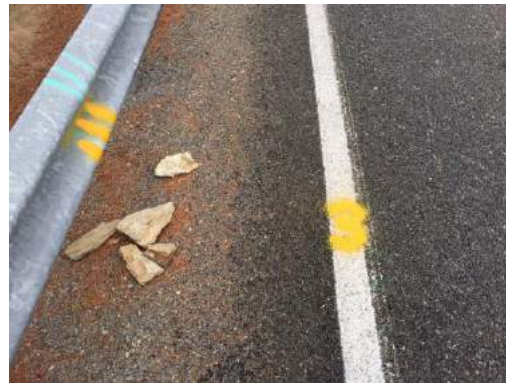
300 metre RSP Road Marking
